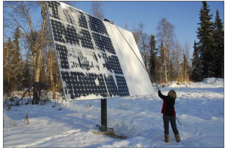
The author's solar panel tracks the midnight sun across the sky, generating power in the process.
